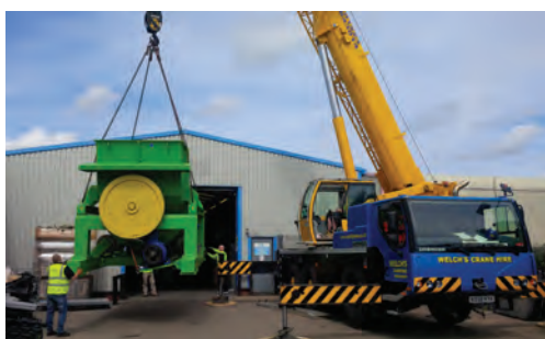
Smash Boom Bang machine being installed at St Ives
